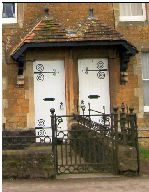
Gates, railings and decorative hinges at Cumnock Terrace
