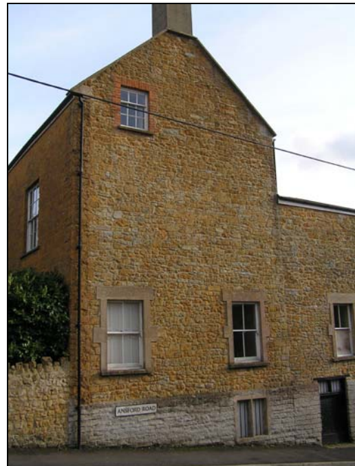
Cary stone ashlar and rubble with Lias plinth
