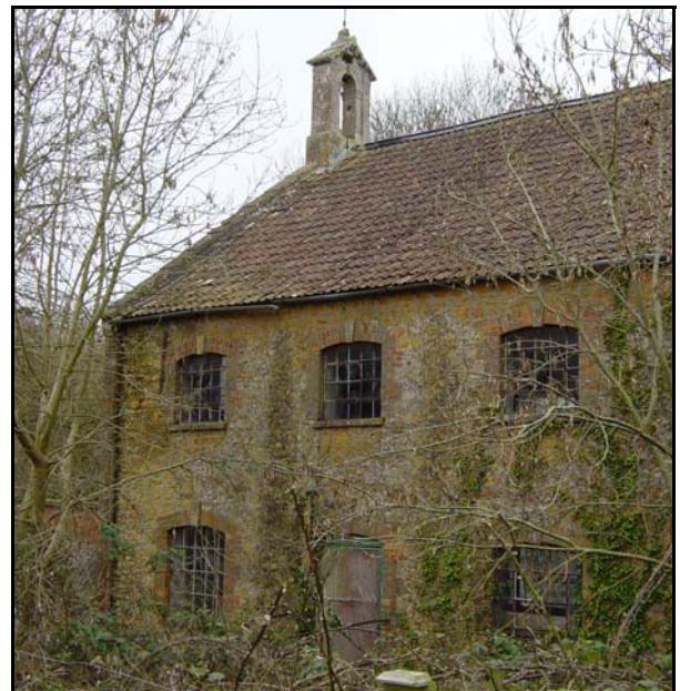
The Flax Mill, needing new uses and repair
