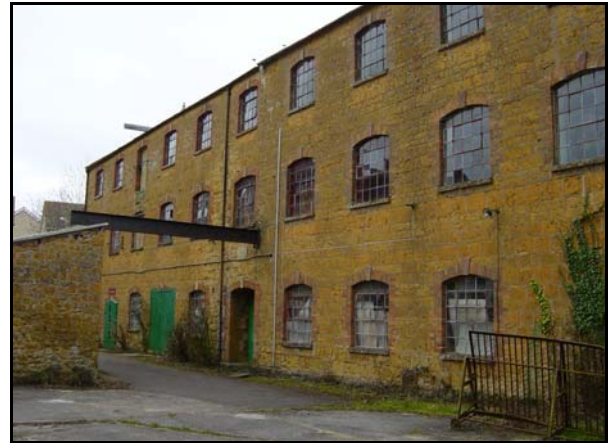
Materials: Flax Mill, Cary Stone & red brick (see drawing at end of report)
