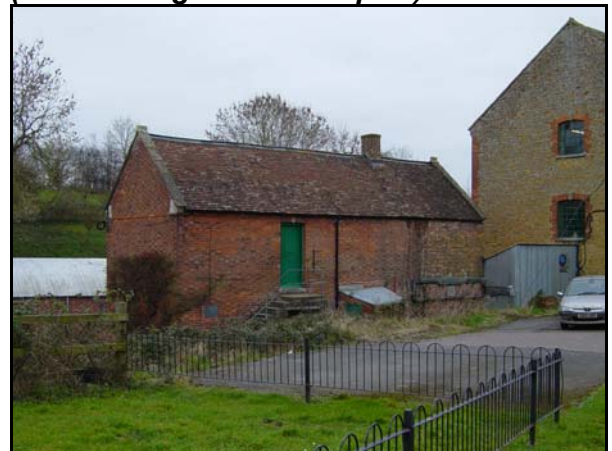
Materials: brick with vitrified headers, Dyehouse
