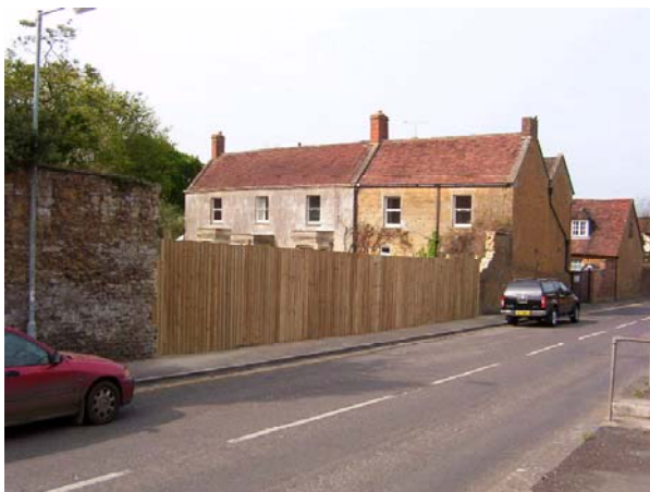
Station Road boundary wall of Millbrook House
