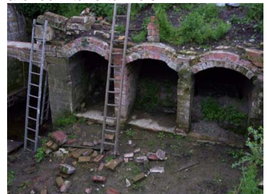
Repairing the entrances to the brick arched intake tunnels.
