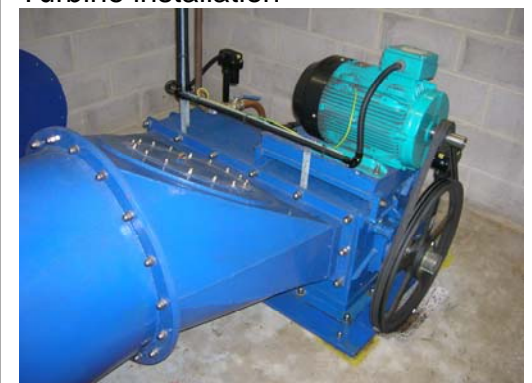
Turbine installation
